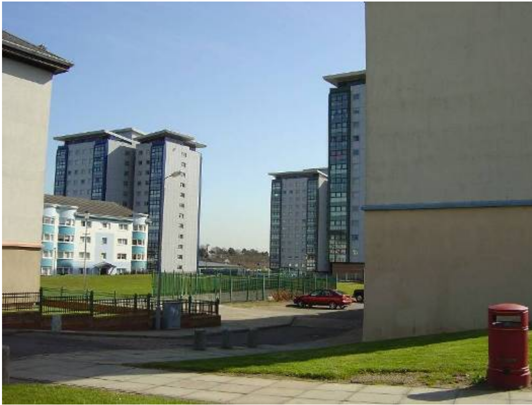
Multi storey and low rise properties after improvement work
