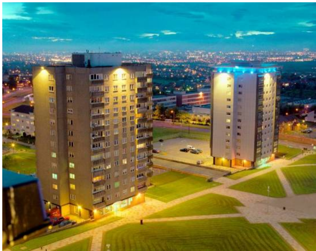
Multi storey blocks before and after improvement
